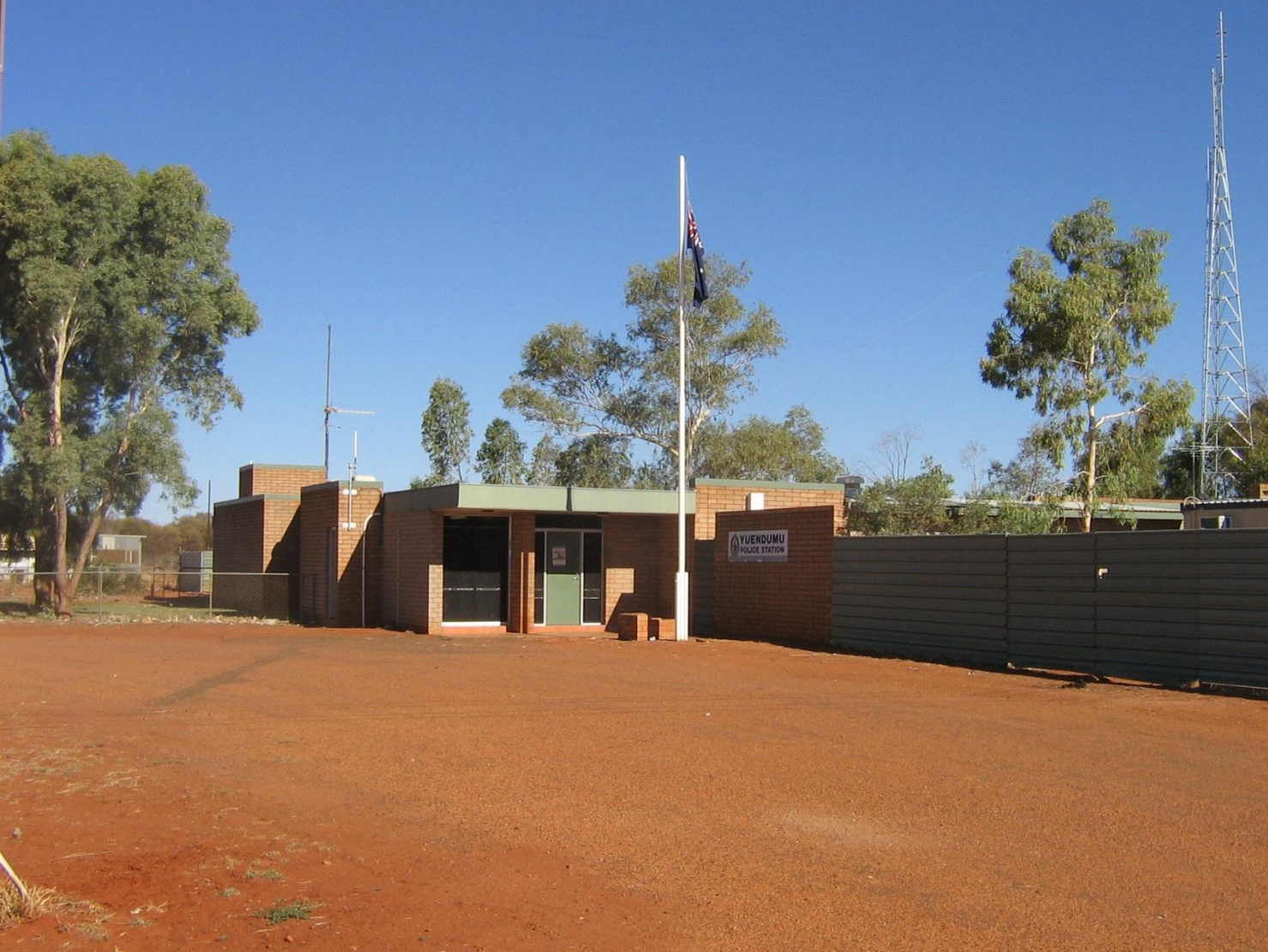
Yuendumu police station
