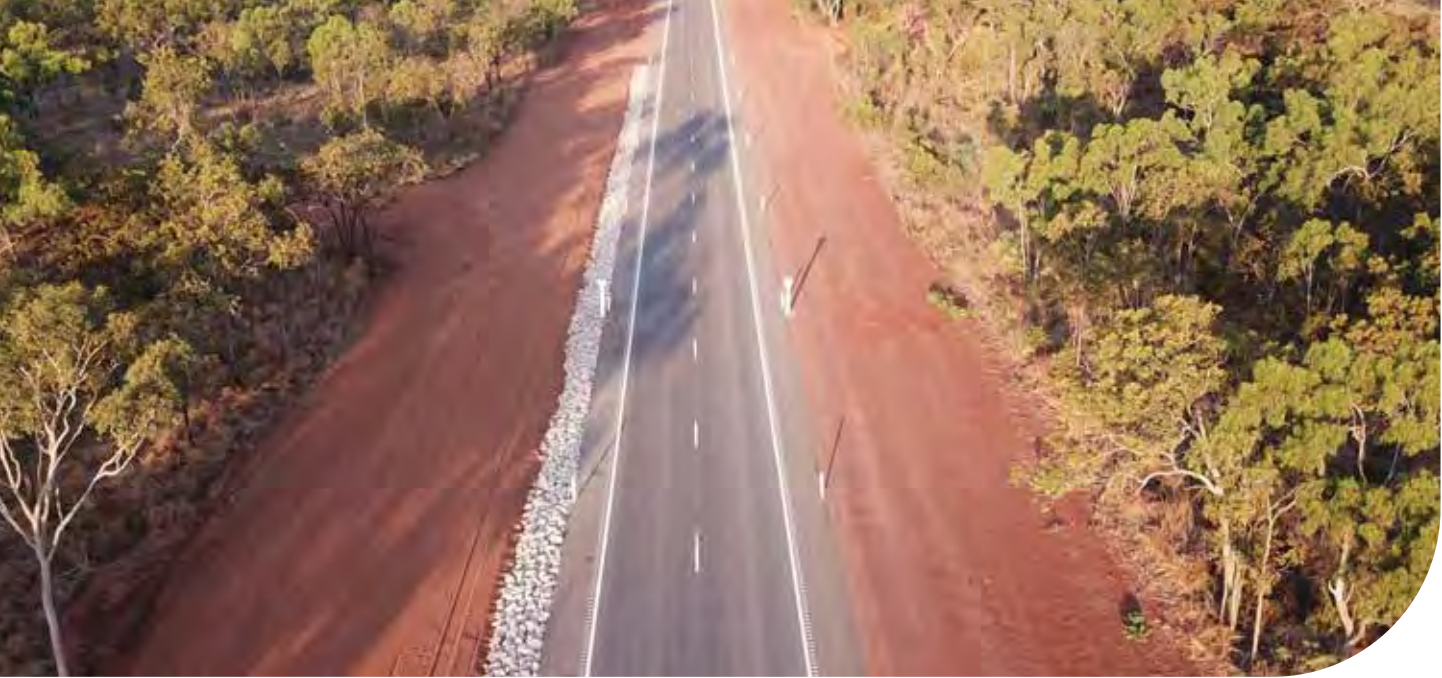
Above: Carpentaria Highway. Credit: Department of Infrastructure, Planning and Logistics.
