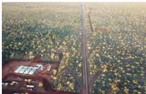
Above: Workers camp for Carpentaria Highway. Credit: Exact Contracting.
